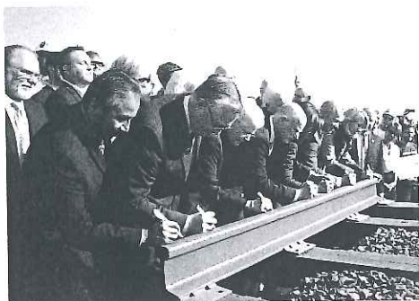
EPA Administrator Gina McCarthy, California Governor Jerry Brown and other officials celebrate the start of construction on the high-speed rail project.
